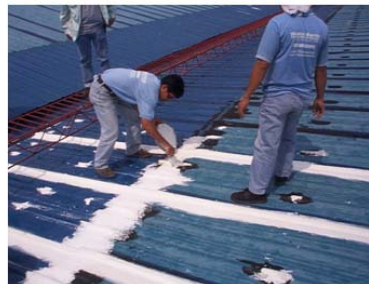
Reinforcement of seams with primer prior to EPDM application
