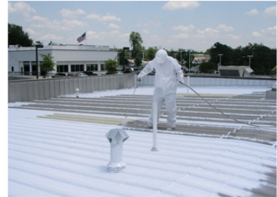
Sprayed application on Corrugated metal
