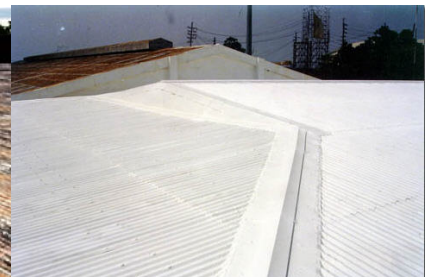
Before and After Picture of Application on Metal with rust. Rust did not need to be removed
