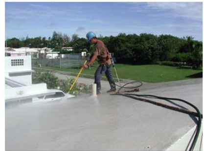
Concrete roof application 25,000 Sq ft area
