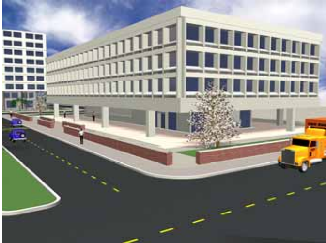
Access denial with anti-ram walls
