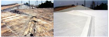
Before and After Picture of Application on Metal with rust. Rust did not need to be removed
