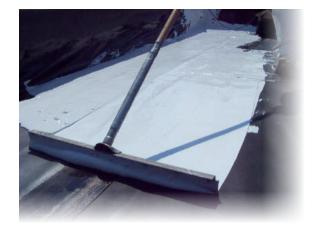
BUTYL TAPE, POLYESTER FABRIC OR BUTYL TAPE-To strengthen damaged roof skin or for reinforcing any worn seams
